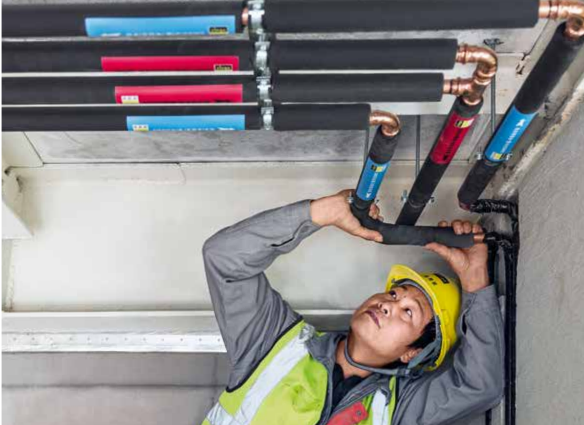
Over 100,000 metres of Viega Profipress copper pipes were installed in the buildings.
